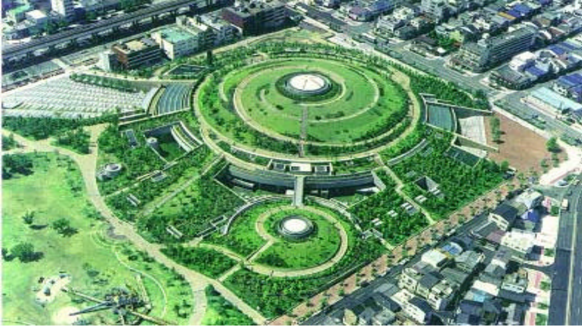
Photo.8 General view of completed work
