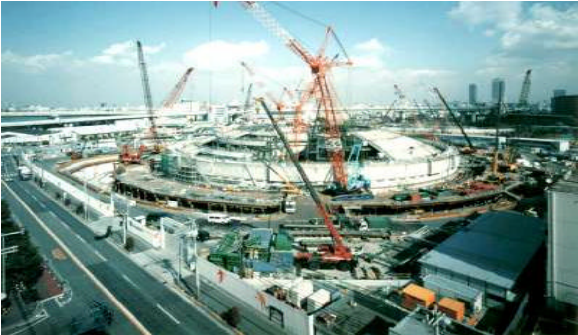
Photo.2 Construction of shell dome
